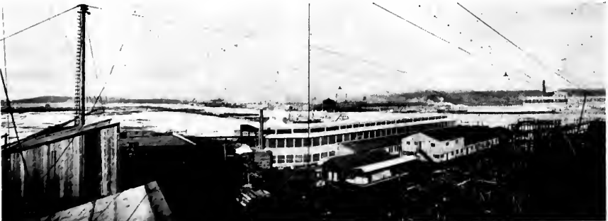
The J. F. Duthie & Co. plant is well laid out for the expeditious handling of steel material between shop and building-ways.
